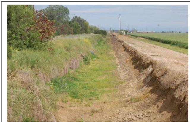
**A section of the water delivery system for the Yolo County Flood Control and Water Conservation District. Vegetated section at left prevents erosion and provides for wildlife habitat, while the section at the right, not vegetation, delivers sediment into local waterways.**
